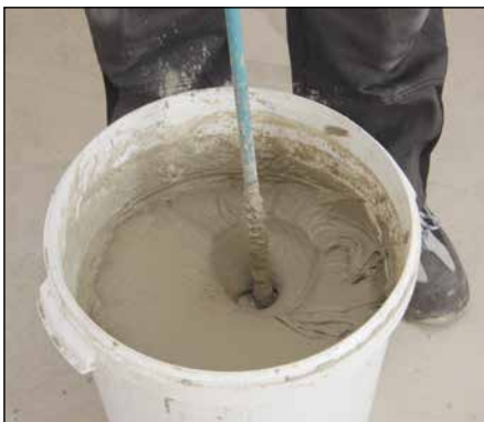
10 Anrühren des Fliesenklebers, z. B. DITRA-X1 made by Sopro.
